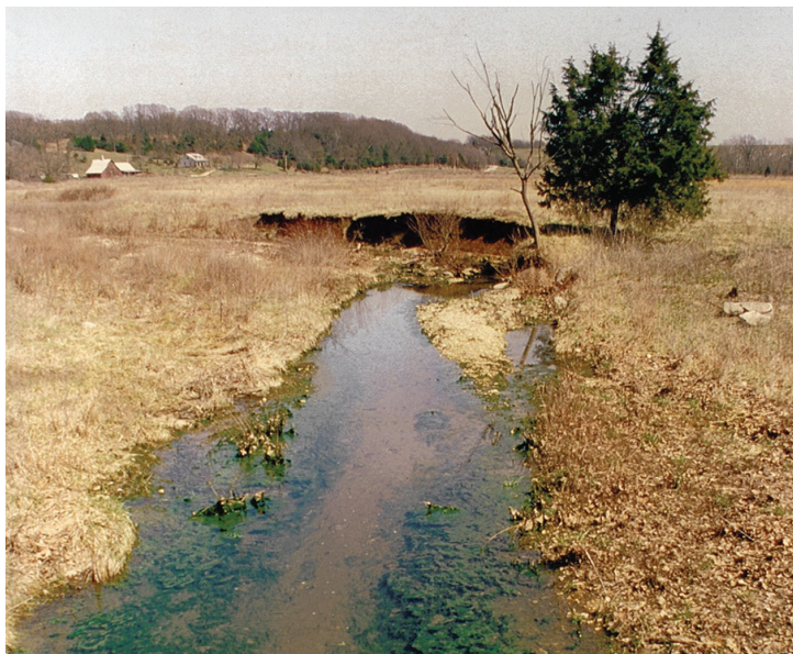
BEFORE: Without a properly stabilized streambank, the stream running through this farmland has eroded the bank and carried valuable soil away.
